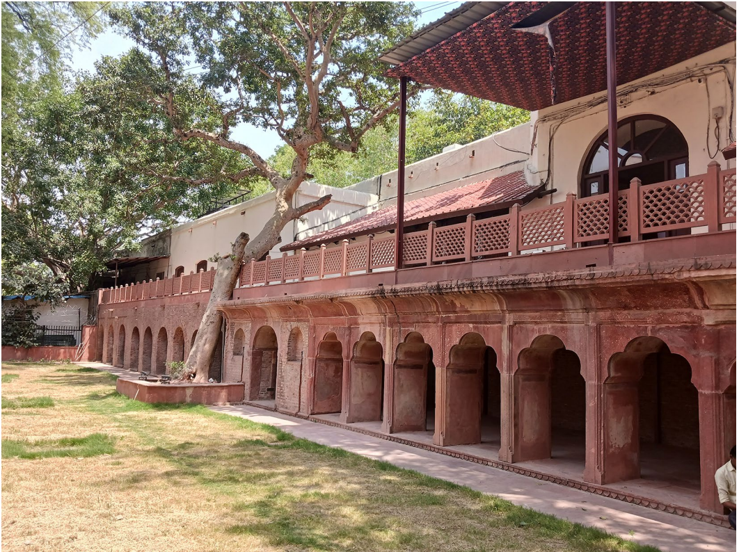
Figure 2. Mughal-styled arches in red sandstone decorate the rear of the library building, New Delhi. Courtesy of the author.
