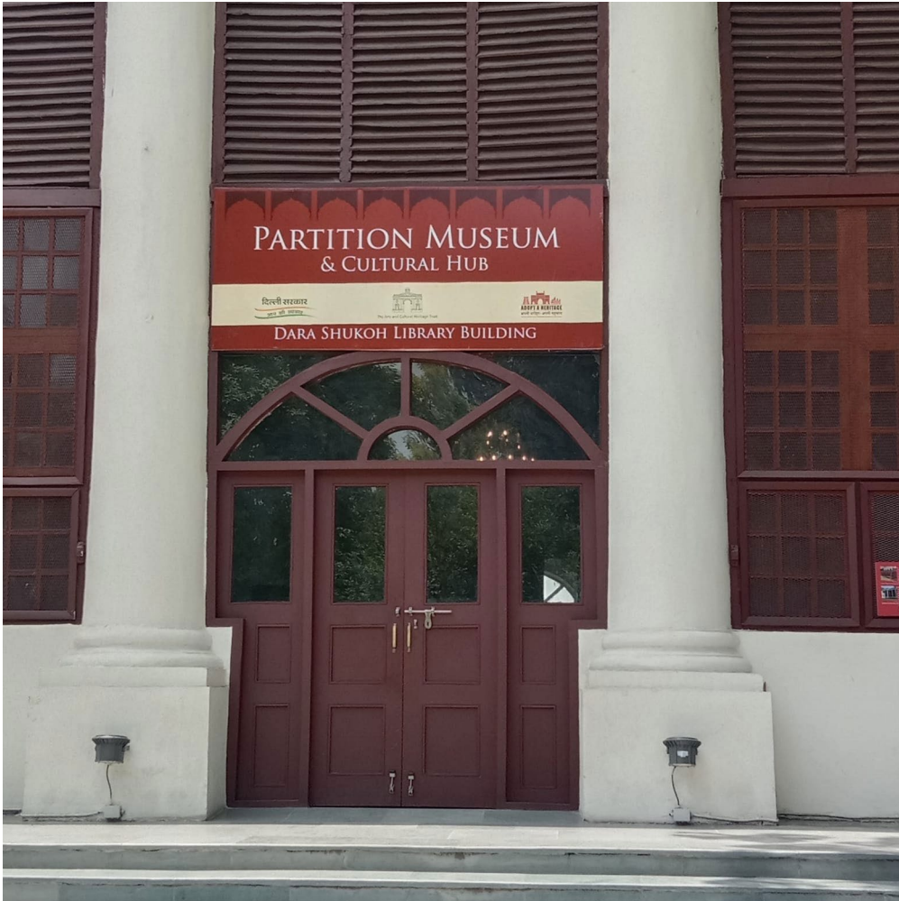
Figure 3. The architectural style of the entrance to the library building contrasts with the Mughal-styled arches, New Delhi. Courtesy of the author.
