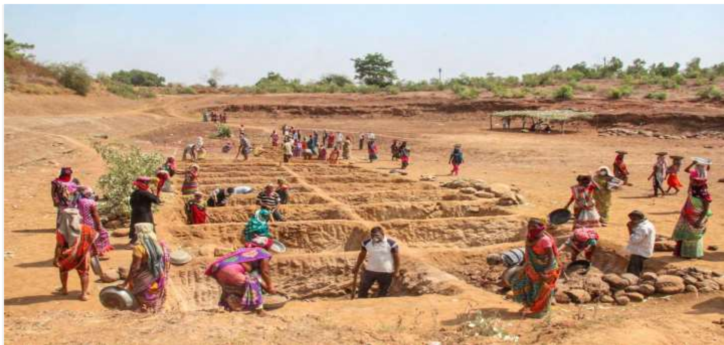
Labourers at an MGNREGA construction site in Navsari. Photo: PTI/File
