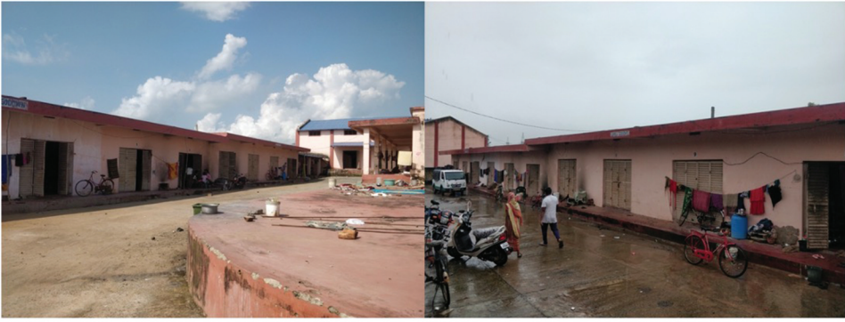
Figure 3. Railway warehouse complex of Meta Sahi (Photos taken by authors).
