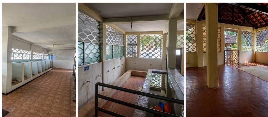
Fig. 7 Spatial additions—Lavatories, new ablution area, front portico (Source: the author)
