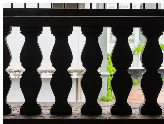
Fig. 15 Detail of decorative balustrade provided in the first-floor veranda (Source: the author)
