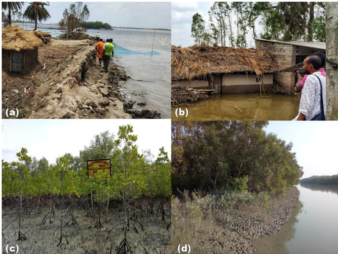
Figure 2: The devastation caused by AMPHAN cyclone at Indian Sundarbans and how mangrove plantation of 2012 acts as a barrier against the vagaries of the supercyclone. (a) The banks and mudflats not protected by mangrove cover have been breached during the cyclone causing extensive flooding across the area inundating agricultural lands. (b) Flooding after the cyclone has inundated many of the houses in the village. (c) Eight year old mangrove plantation ( Rhizophora mucronata ) along the mudflat of the river banks of Lahiripur Gram Panchayet (village). (d) Mangrove cover grown due to the plantation activity of 2012 has protected the village from AMPHAN by stabilizing the mudflats.
