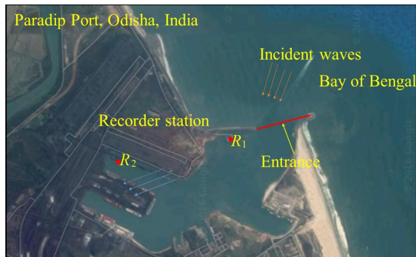
FIGURE 4. Bird view of the Paradip port, Odisha and two record stations are considered as R_1 and R_2 and red arrows show the incident waves propagating toward harbor's entrance.
